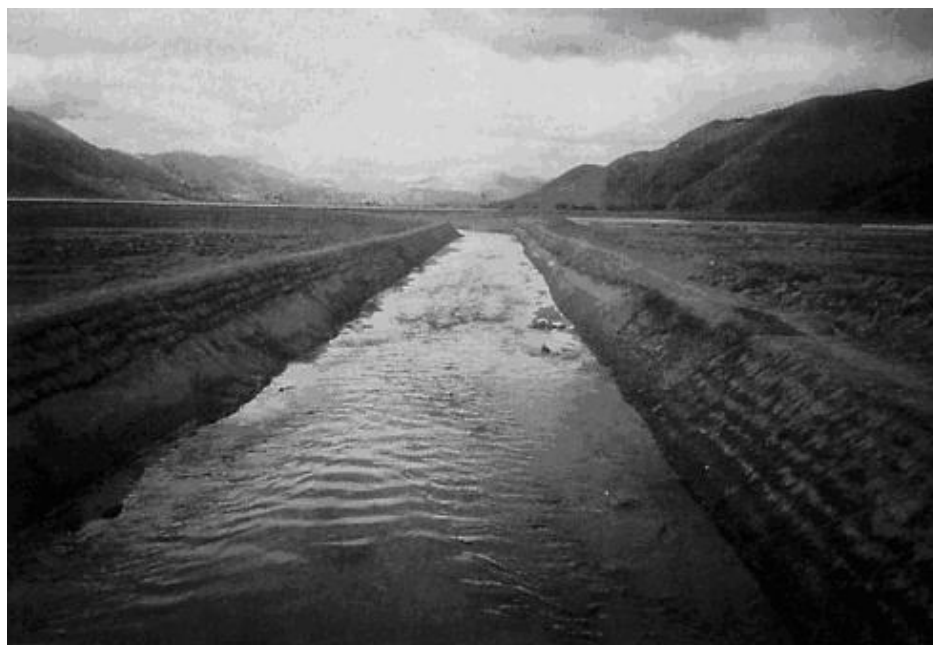
Photo 10. A brook, traversing the pampa (a former lake filled with sediments) has been bunded with sods (champas) from the surrounding natural pastures, an effective way of flood-control.
