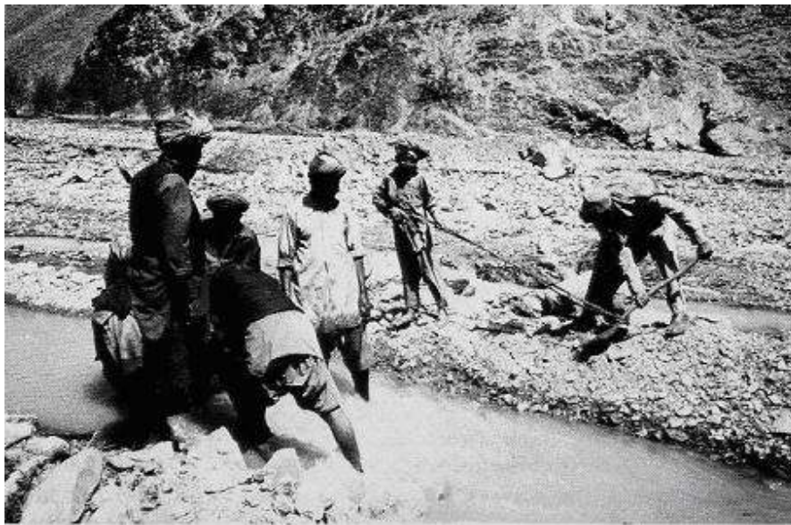
Photo 3. Reconstructing a traditional diversion weir
