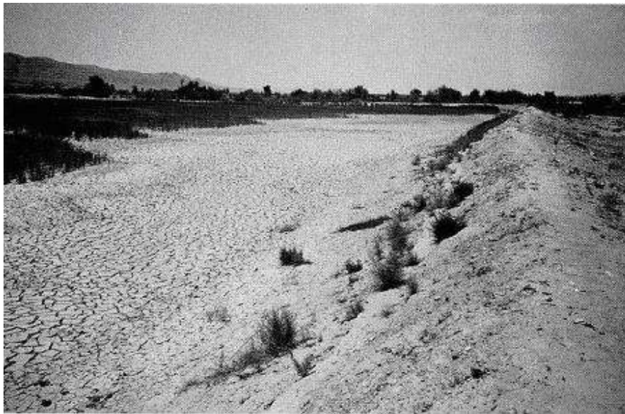
Photo 1. Earthen bund for water harvesting
