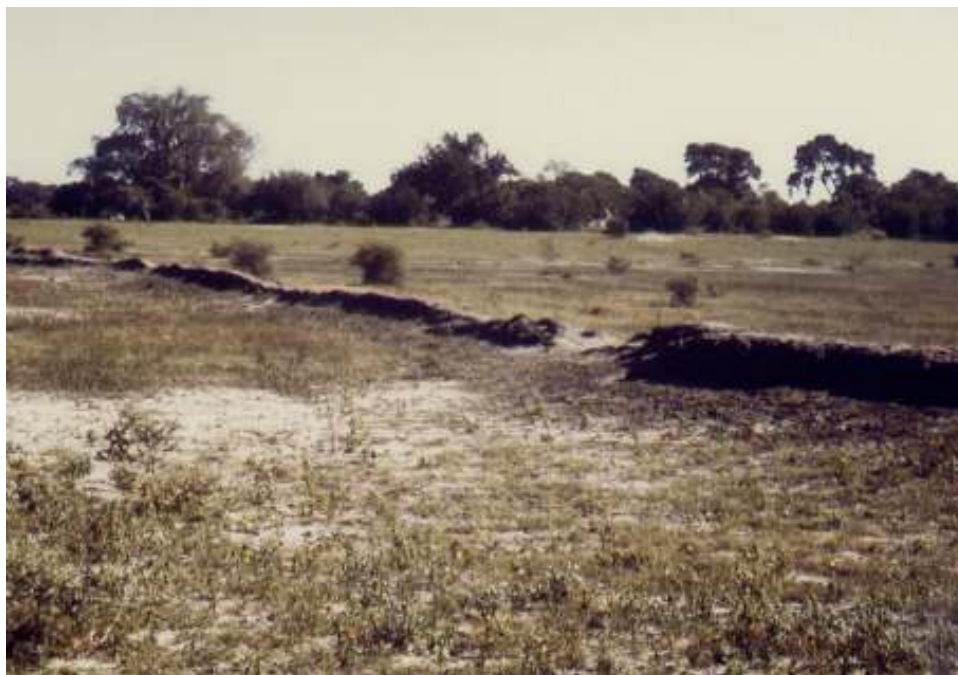
Old, abandoned traditional bund made to retain water in the molapo for flood-recession cropping
