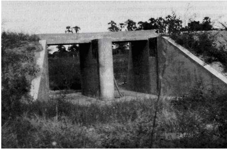
Photo 6. Close up of the sluice gate of the bund in Photo 5.
