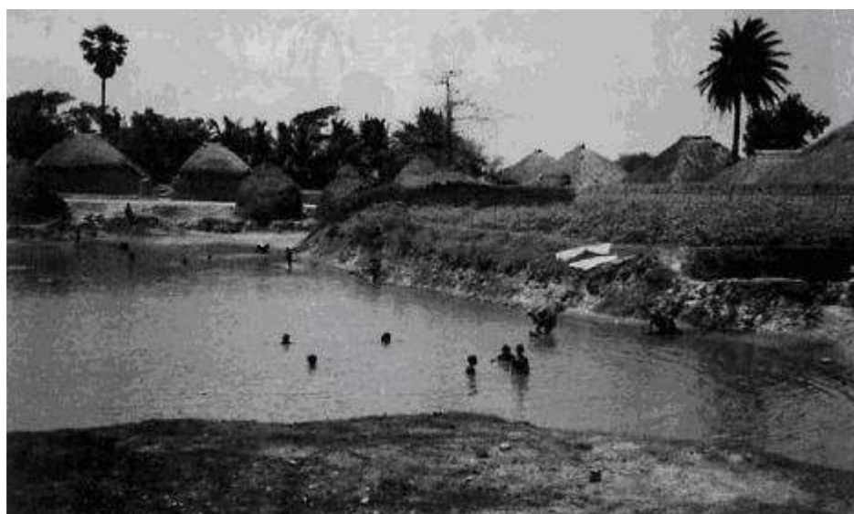
Photo 4. An excavated natural creek serves as a village pond and stores water for domestic purposes, the irrigation of Rabi crops, and fish culture.
