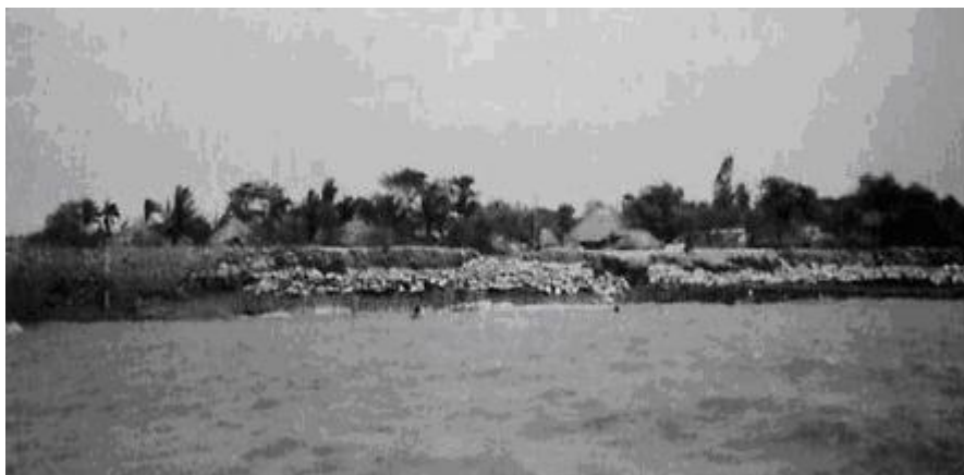
Photo 2. Showing one of the Matla river, on of the many large tidal estuaries. Note the decay of the protective bunds.
